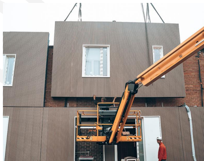
Figure 36. Installation of prefabricated wall elements on site, by BuildUp Offsite Company, https://www.buildupoffsite.com/nl_BE/about-us/our-story . Copyright by BuildUp.
