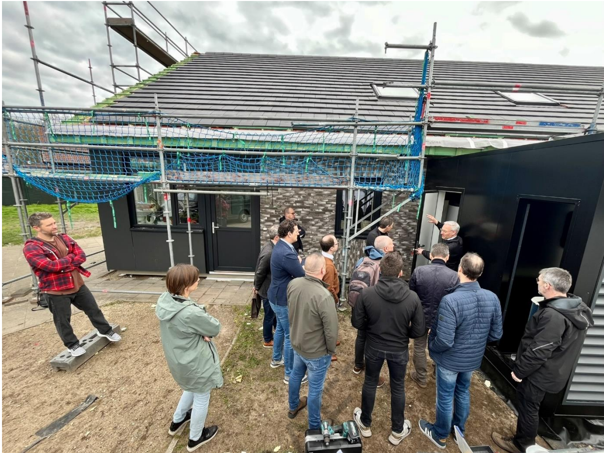
Figure 13: Visitors of renovated dwelling inspecting the energy box
