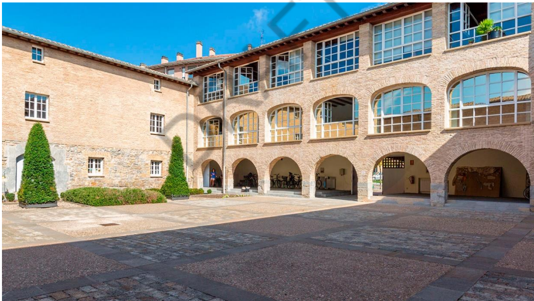
Figure 16: Headquarters of the Positive Energy District Office in Pamplona
