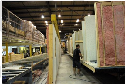
Figure 14: Example picture of prefabrication 34
