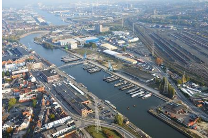
Figure 11: Example of Flux50-supported project: De Nieuwe Dokken
